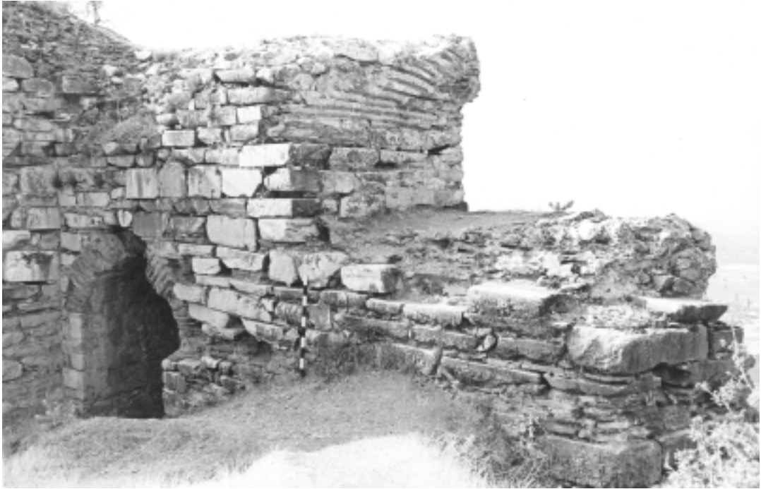
2. Sardis. Entrance into the Byzantine fortifications on the acropolis, showing masonry taken from earlier buildings. Courtesy of the Archaeological Exploration of Sardis/Harvard University (70.211:36a)
